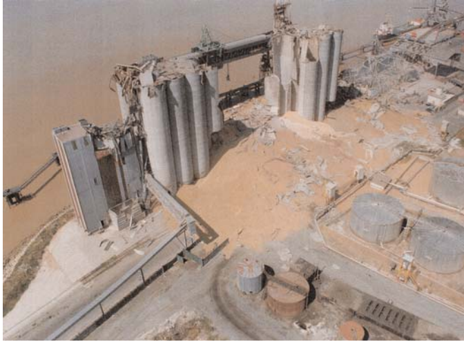
FIG. 1—The silos in Blaye after the explosion.
